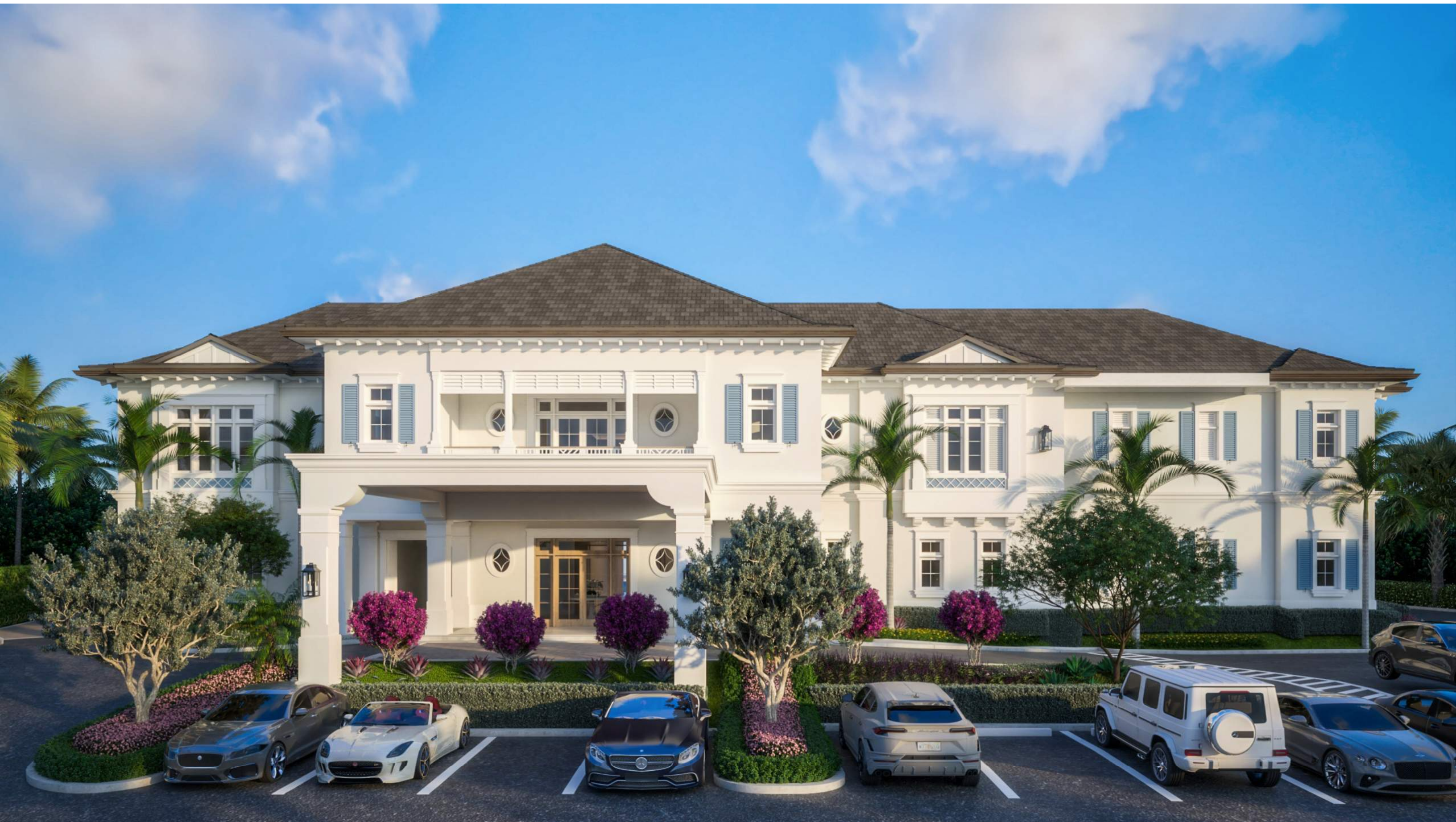
Front Elevation (Looking East)
