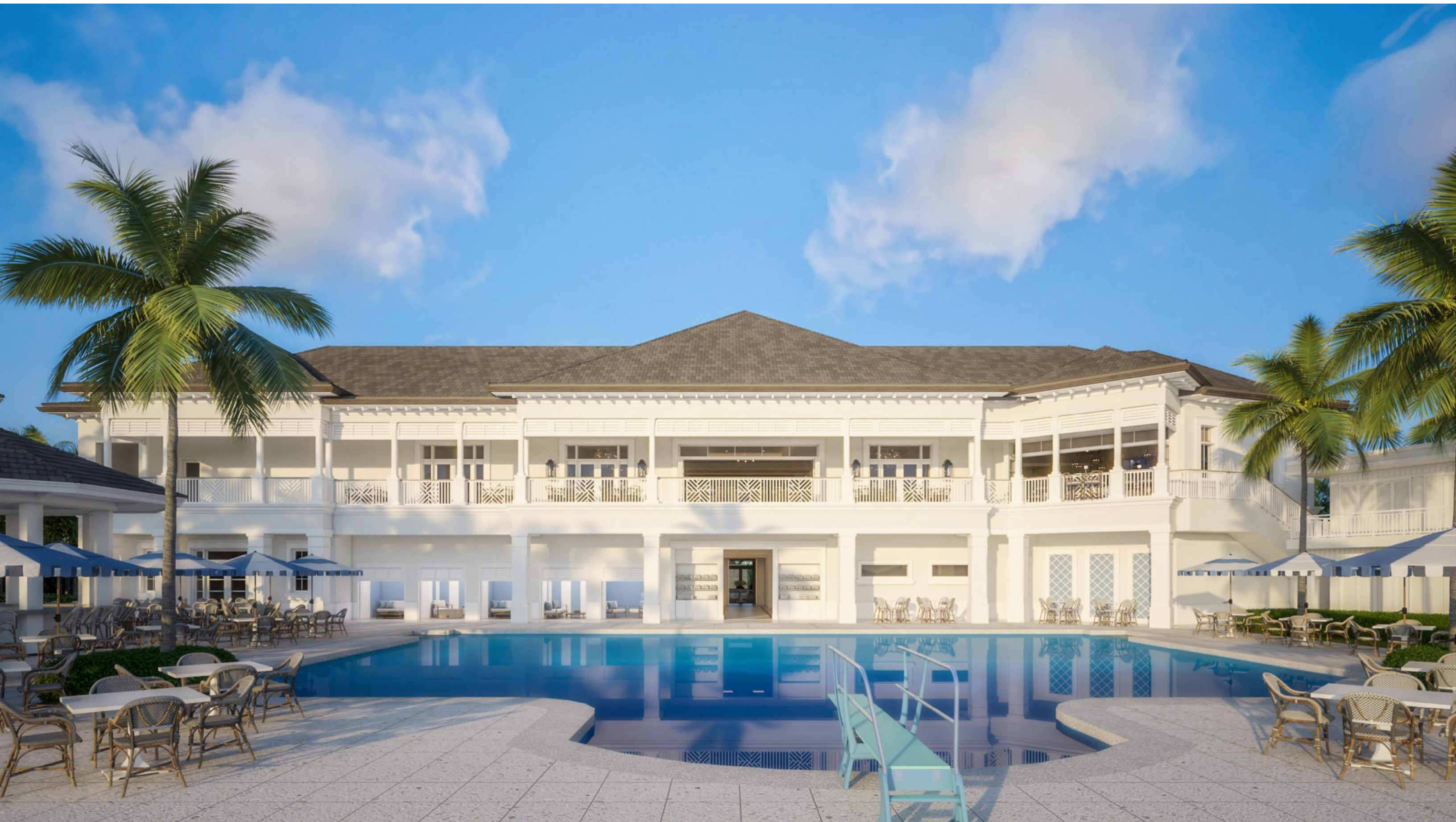
Rear Elevation (Looking West)
