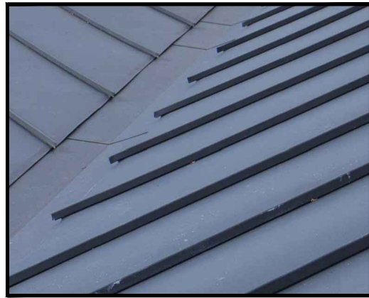
STANDING SEAM METAL ROOF DARK GRAY
