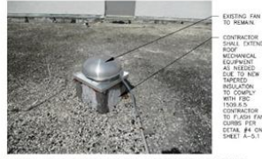
BB1 TYP. ROOF FAN FLASHING PHOTO
