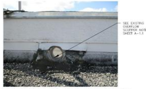
FF1 TYP. SCUPPER AT CURVED WALL PHOTO
