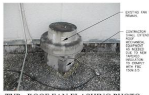
BB1 TYP. ROOF FAN FLASHING PHOTO
