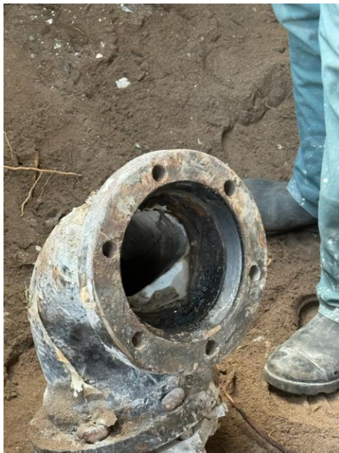
Figure 3: Removed 90 degree bend
