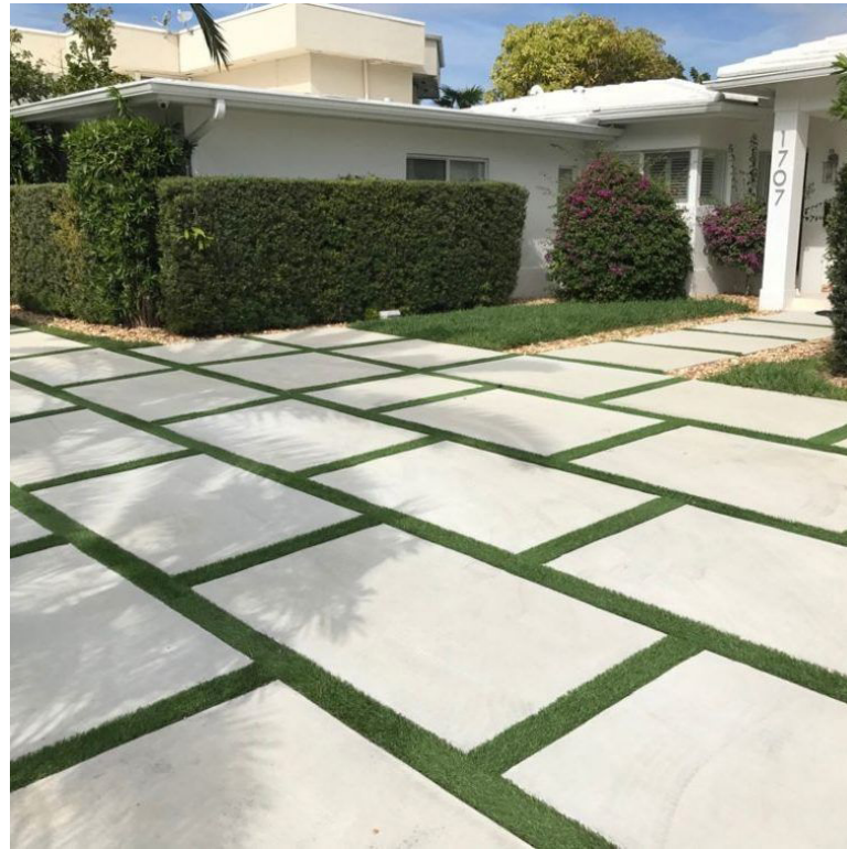
Concrete driveway with turf joints
