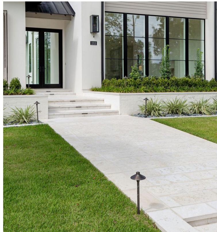
Paver entry walkway
