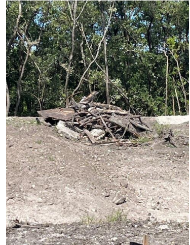
Debris piled up on site
