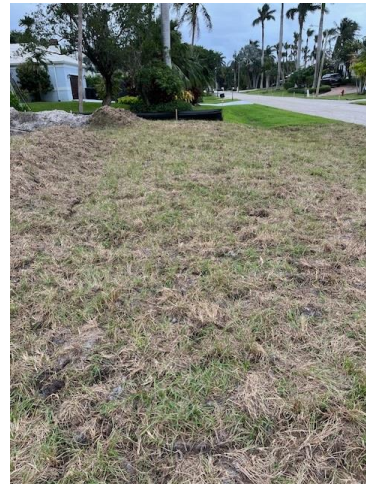
Right-of-way roughly graded
